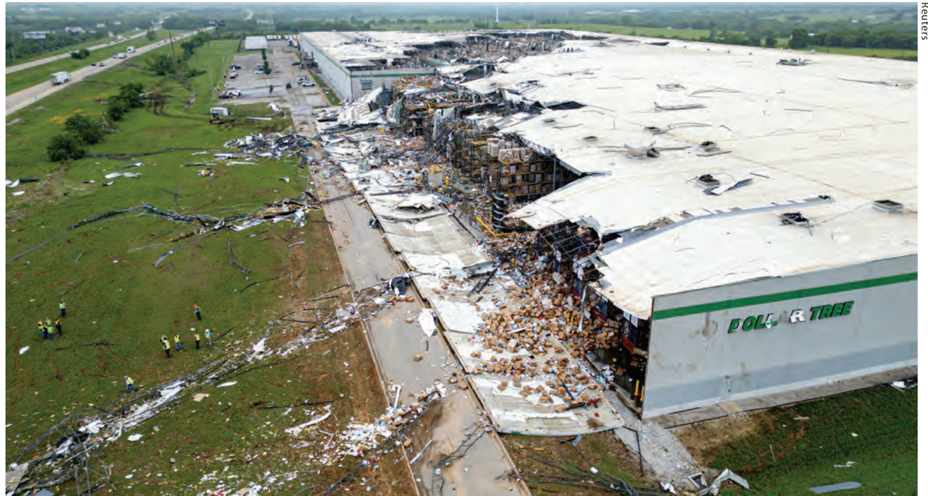
A Dollar Tree warehouse in Marietta, Oklahoma, was severely damaged by a tornado in April.
