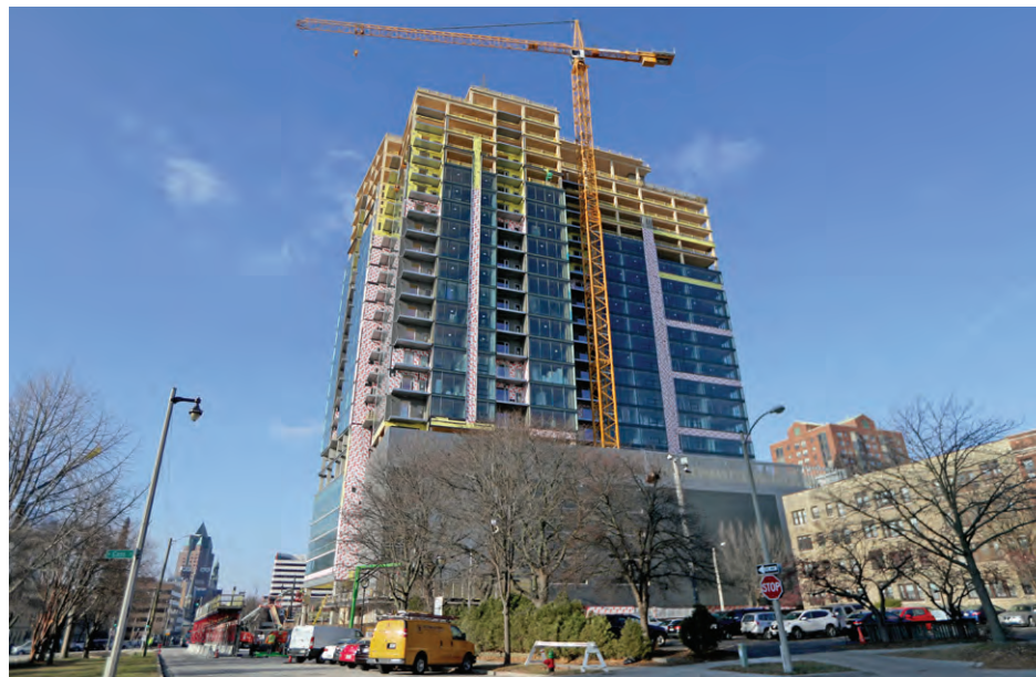
The Ascent, a 284-foot, 25-story apartment building under construction in Milwaukee is described as the tallest mass timber structure in the world.
